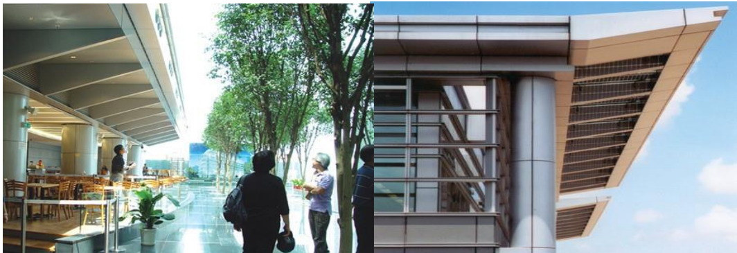
Figure 2.1: Hong Kong Science Park – Solar Glass (Source: www.google.com )
